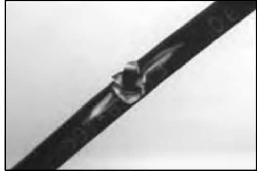
Inspect air line for holes and cracks. Replace as needed.
